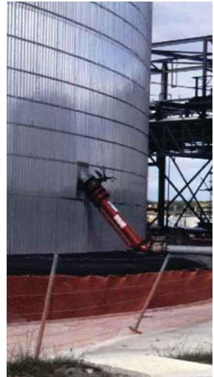
Example of sub-surface foam application apparatus
